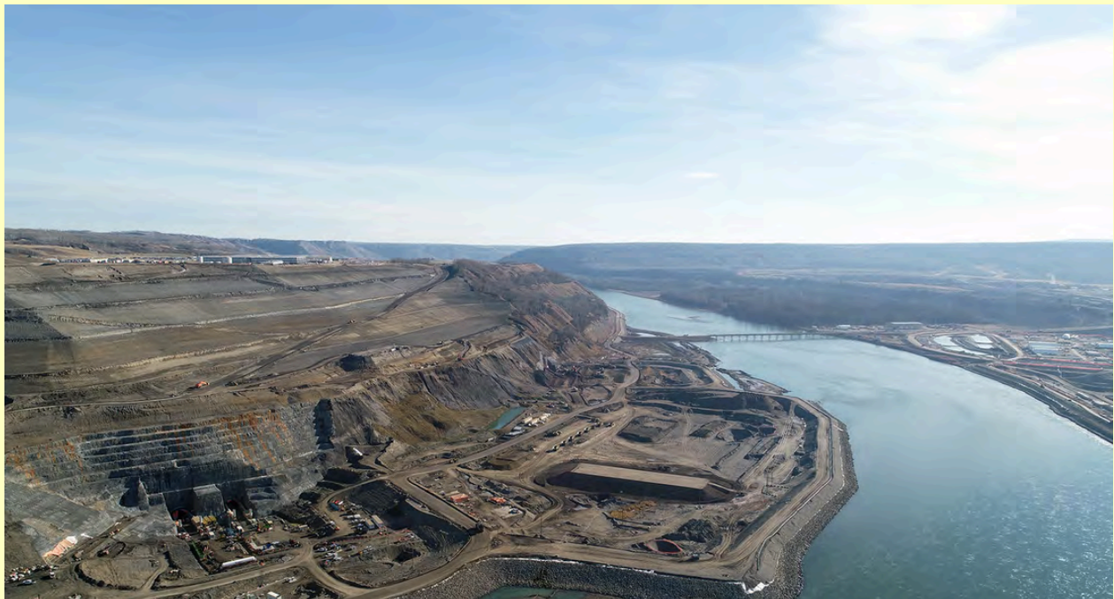
North bank, looking downstream (October 2018) Photo: BC Hydro
