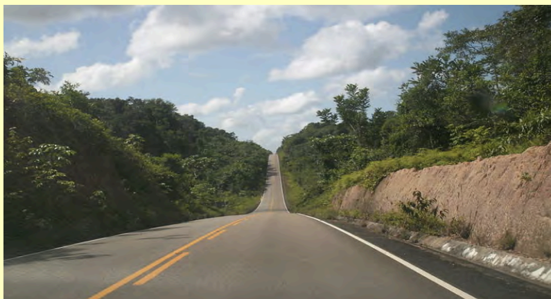
The BR-174 where it runs through the Waimiri Atroari Indigenous Reserve. The transmission line, if built, would run beside it. Construction is slated to start in June, though could be delayed by a court challenge. Image by SallesNeto BR licensed under the Creative Commons Attribution 3.0 Unported license. (Rocha, 2019)
